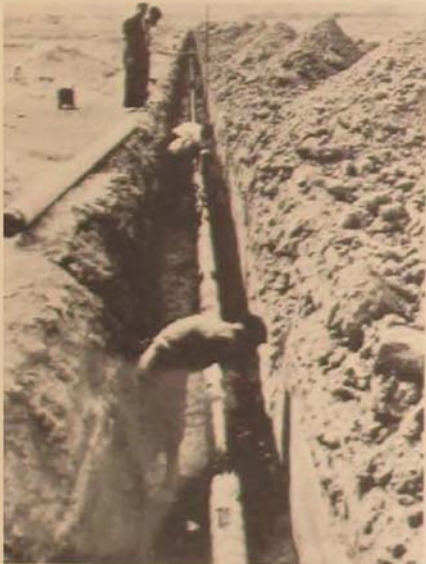
. . . lay fuel pipelines,
